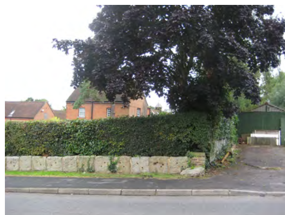
Picture 9.9 Boundary treatment to Pinner Hill Farm
