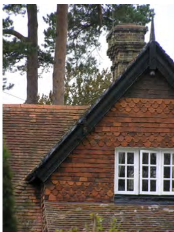
Picture 9.17 Gable ends
