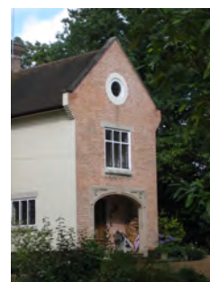
Picture 9.27 Stone lintels
