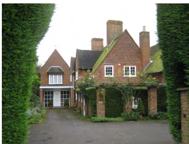
Picture 9.19 Steeply pitched roofs
