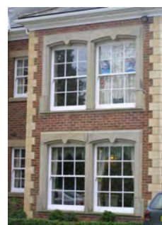
Picture 9.36 Stone quoins and window surrounds
